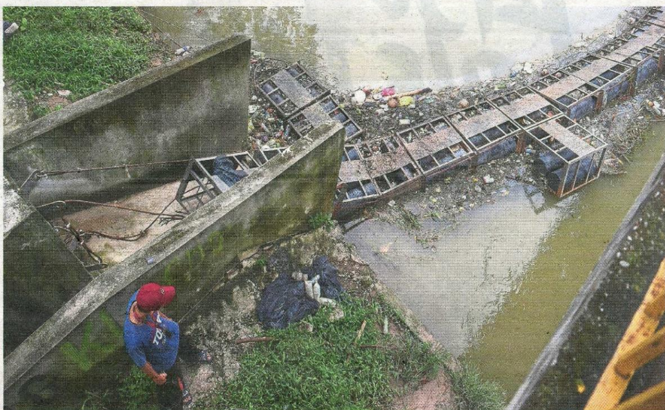
The human stain: A debris trap in Sungai Gombak, which was part of the River of Life project to rehabilitate waterways and part of the Greater Kuala Lumpur project that began in 2011. — Bernama
